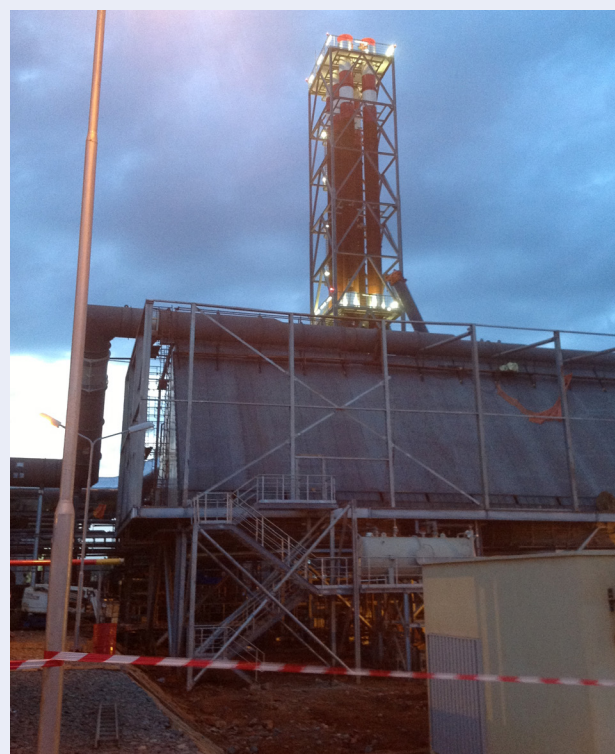
Thika power plant during construction.
